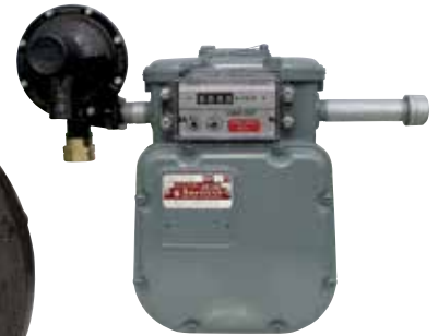
Attached to Vapor Meter
